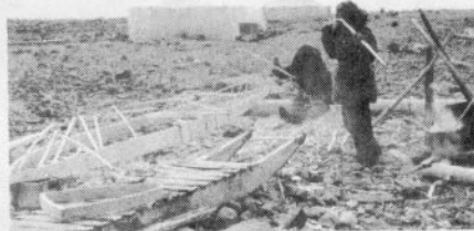
FIGURE 3: HULL RIBS ARE SOAKED IN BOILING WATER TO EASE BENDING.
